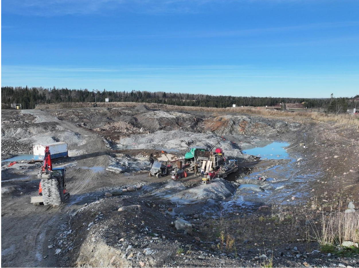
Figure 3: Keats excavation grade control drilling.
