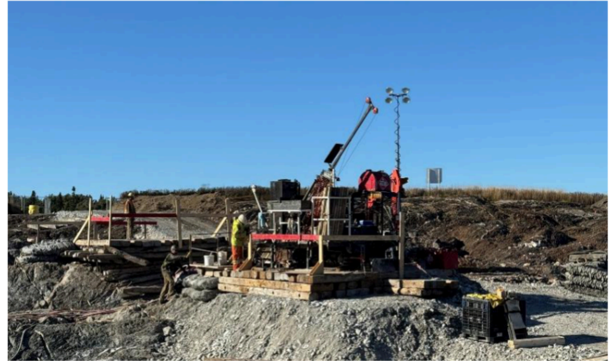
Keats Excavation: Grade Control Drilling
