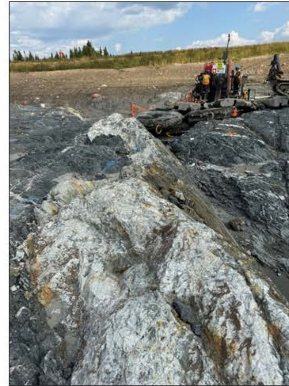
Grade Control Drilling in Keats Excavation
