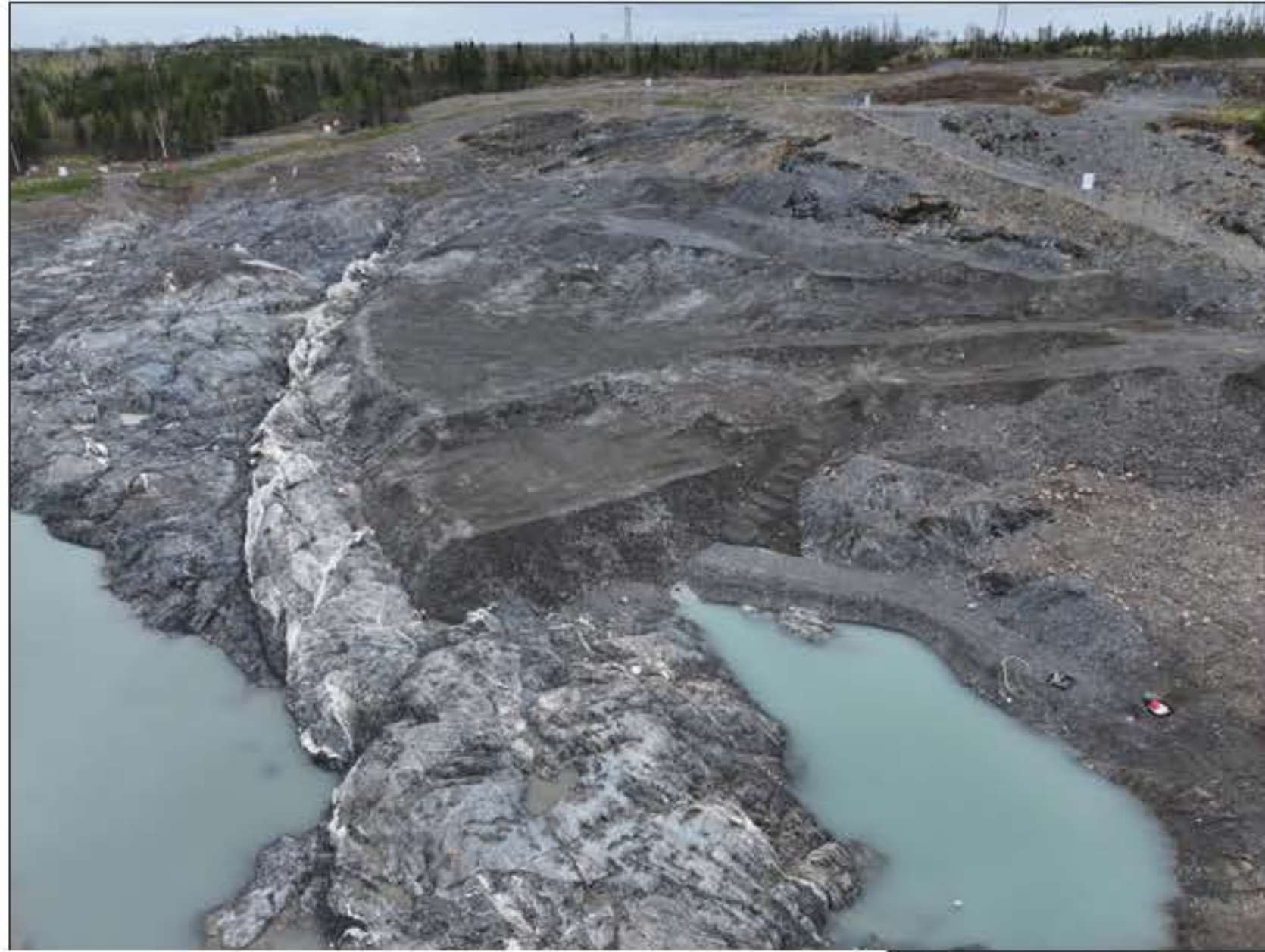
Iceberg grade control pad development
